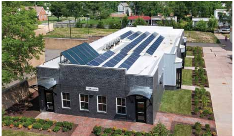
Somanath Senior Apartments at Beckstoffer's, the first projected net-zero energy apartment building constructed in Virginia, brings high performance housing to low-income seniors in the Church Hill neighborhood of Richmond. Seven one-bedroom/one-bath units averaging 700 square feet feature mini-split ductless heating and cooling systems, energy recovery ventilation devices, and harvest energy through both photovoltaic panels to produce electricity and solar thermal panels to produce hot water.
